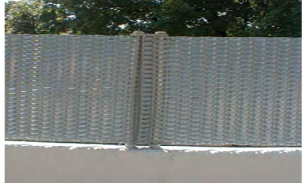
7. When joining two rolls of DRC Fabric, use the splice plates provided (See drawing for anchor locations at splices). Insert the  $\frac{3}{4}$ " post bolt through the splice plate first and then through the DRC Fabric.
