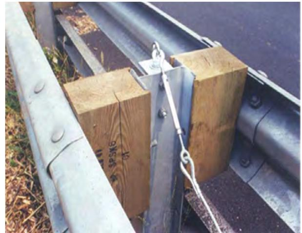
9. Loop the Cable Anchor Assembly over the last  $\frac{3}{4}$ " bolt in the run of fabric. Then attach the Cable Anchor Assembly to the angle bracket using the  $\frac{3}{4}$ " eye bolt. Place one nut above the bracket and one below and tighten. Tighten the  $\frac{3}{4}$ " turnbuckle until the DRC is taut.
