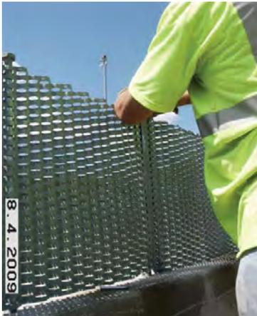
Next insert the second  $\frac{3}{4}$ " post bolt through the same splice plate and then through the "new" roll of DRC Fabric in the first row beyond the starter tab. Attach the post bolt to the angle bracket as shown, using a nut above and below the angle bracket. Re-attach the come-a-long to the opposite end of the DRC Fabric.
