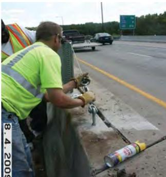
Tighten the  $\frac{3}{4}$ " turnbuckle finger tight. See attached detail drawing.
