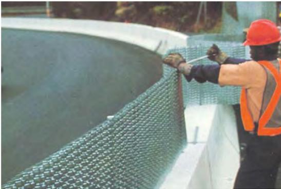
2. Insert  $\frac{3}{4}$ " Post Bolt through the first row of DRC Fabric and attach the End Treatment Cable Anchor Assembly to the top of the  $\frac{3}{4}$  Post Bolt as shown in the detail drawing. Insert the threaded end of the post bolt into the second anchor location. Secure Cable Assembly using  $\frac{3}{4}$ " eye bolt attached to the first expansion anchor in concrete barrier.
