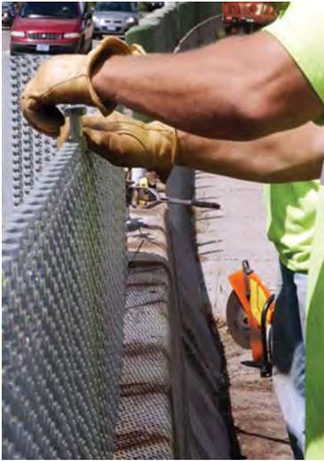
6. Continue to insert  $\frac{3}{4}$ " Post Bolt through the DRC Fabric at the anchor locations. Use the come-a-long to position the bolt over the anchor, keeping the DRC fabric taut.
