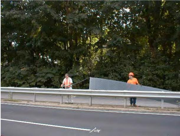
7. When joining two rolls of DRC Fabric, use the splice plates provided. Insert the  $\frac{3}{4}$ " post bolt through the splice plate first and then through the DRC Fabric. Secure the bolt to the two-hole splice angle bracket as described in Step 3. Trim the fabric and leave one row of fabric beyond the post bolt when trimming. Detach the come-a-long from the remaining piece of DRC Fabric.
