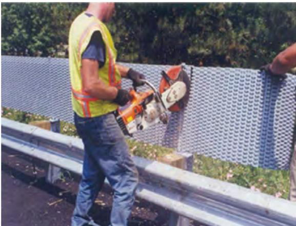
8. Secure the bolt in the anchor and trim the fabric. Leave one row of fabric beyond the post bolt when trimming. Detach the come-a-long from the remaining piece of DRC Fabric. Next insert the second  $\frac{3}{4}$ " post bolt through the same splice plate and then through the "new" roll of DRC Fabric in the first row beyond the starter tab. Re-attach the come-a-long to DRC Fabric.
