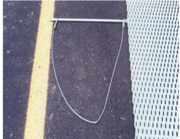
3. Attach the Come-A-Long Cable Assembly provided by Transpo to the opposite end of the DRC Fabric using the  $\frac{3}{4}$ " steel post provided. Please note: Do not use Post Bolt.
