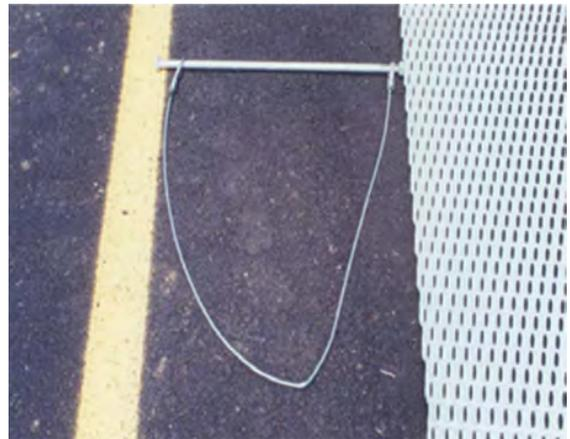
4. Attach the Come-A-Long Cable Assembly provided by Transpo to the opposite end of the DRC Fabric.
