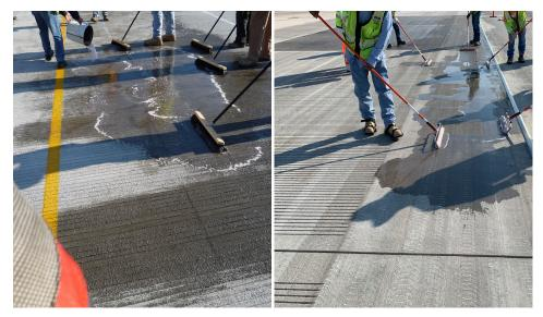
T-78 Polymer Crack Sealer seals cracks effectively and can be open to traffic in *as little as an one hour.*
