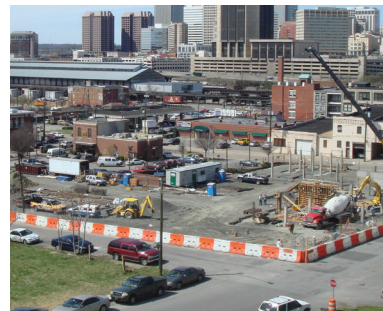
Construction Site Containment
