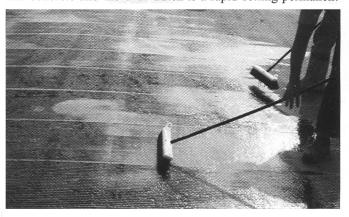
polymer concrete. T-70 Sealate seals concrete cracks in bridge decks, on airport runways and in parking garages. T-48 Chip Seal is easy to apply, waterproof and highly skid resistant.
